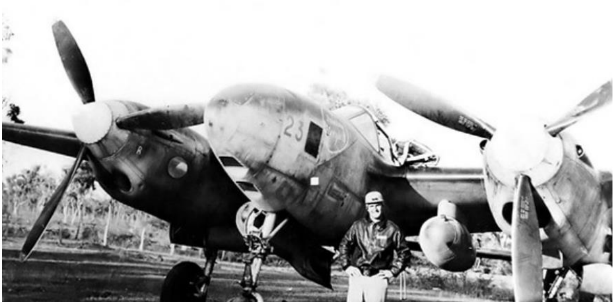
The 8 th Figure 7 - 1942 - An 8th Photo F-4 P-38 Lightning at '14-mile' Schwimmer Airfield complex near Port Moresby. The two vertical camera ports (K-18 24-inch forward and K-17 6-inch closer to the nose wheel) and the port side K-17 oblique camera port next to '23'. In November 1942 this F-4 crashed on take-off killing the pilot.
