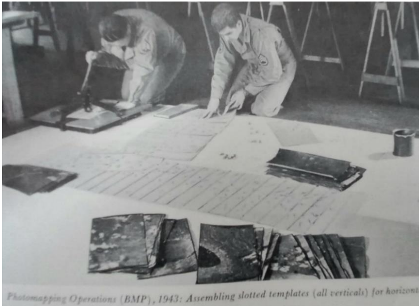
Figure 6 – At US 648 th Engr Topo Bn BMP Melbourne, K-18 24-inch focal length vertical camera large format photographs (9x18-inch) here being used for a slotted templet assembly to establish photo control for mapping likely areas of intensive land combat operations and for targeting.
